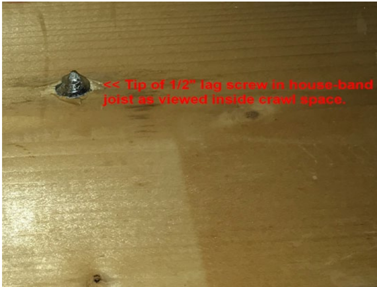
Figure 3. The tip of the lag screw depicted meets the IRC requirement for fully extending beyond the inside face of the band joist.
